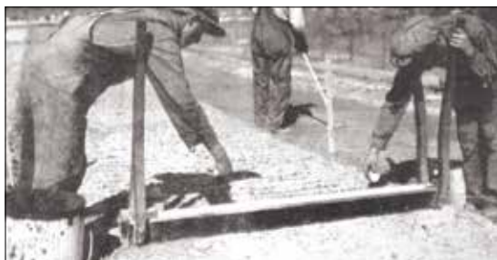
F.O. BATEMAN'S seeder for sowing longleaf pine seeds in the nursery in operation. This simple tool significantly improved the quality of nursery longleaf pine seedlings.
